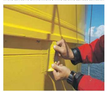
start in many different areas – monopiles, ladders, walkways, boat landings, guard rails and rotor heads – each of which can compromise the overall integrity of the structure. Protective coatings that can be applied to prevent corrosion from developing, or halt its progression, are essential to providing long term asset protection.
